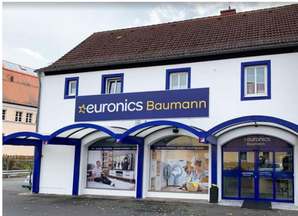
Telekom Partner Baumann GmbH Hauptstraße 75, 91257 Pegnitz
